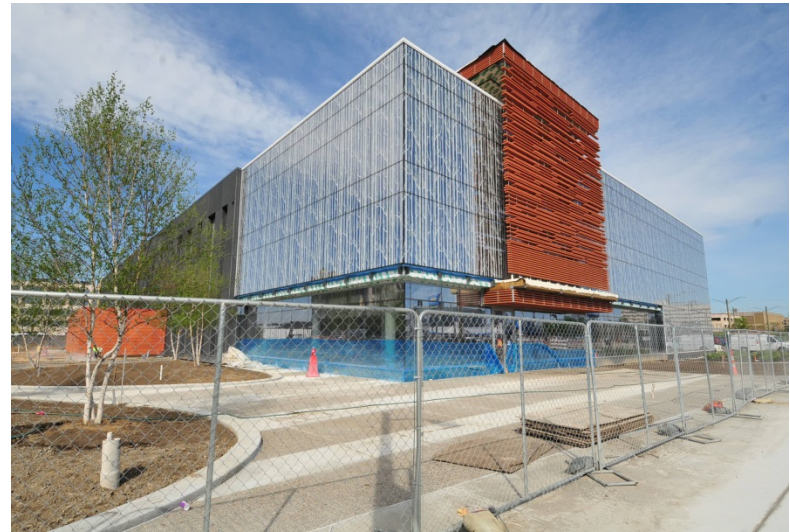
IBio southeast exterior corner
